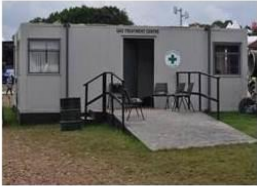
Gas treatment centre
